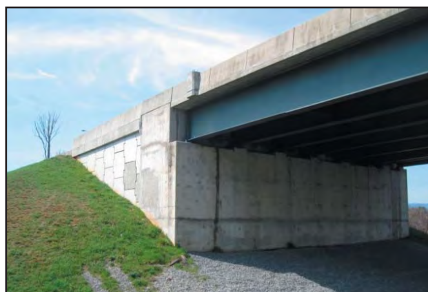
The MSE walls will be set back from the front face of the abutment, similar to the appearance of the existing bridge.
